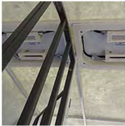
Dual roof vents
