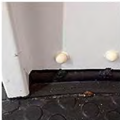
All rivets are rubber backed
